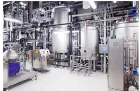
a structure for Application - Fuel Gas Transmission
