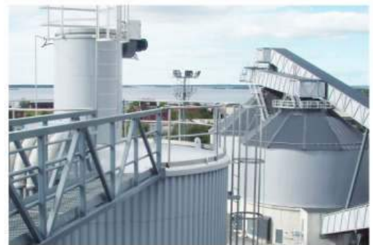
a structure for Application - Ash Handling Plant
