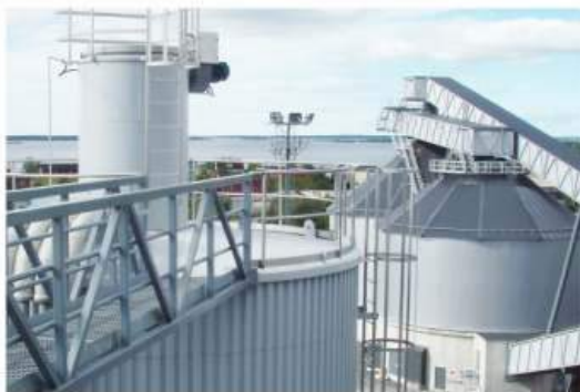
a structure for Application - Ash Handling Plant
