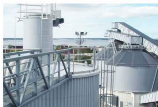
a structure for Application - Ash Handling Plant
